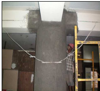
Fig.3 Surface grinded and prepared for fiber wrapping
