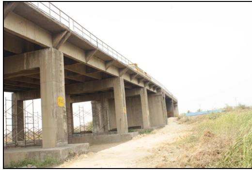
Fig.11 JNPT Rail over bridge at Karal
