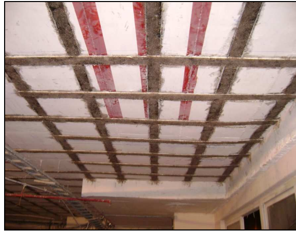
Fig.10 Slab after strengthening by carbon fibre laminates
