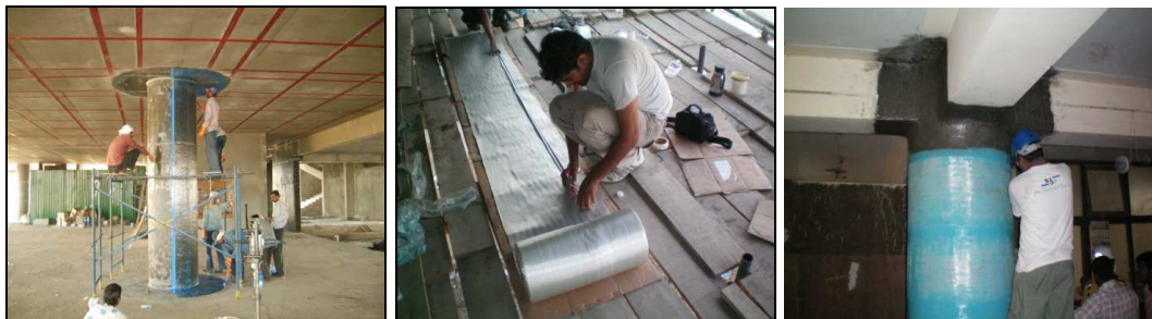
Fig.5 Cutting and applying of fiber sheet on the column
