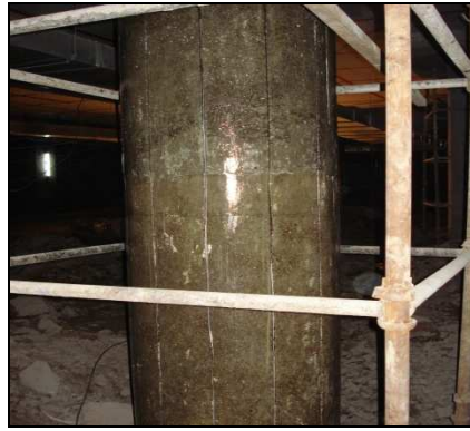
Fig.4 Surface Primer applied on the column
