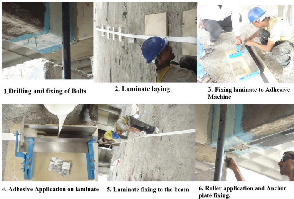
Fig.24 Laminate fixing on the beams
