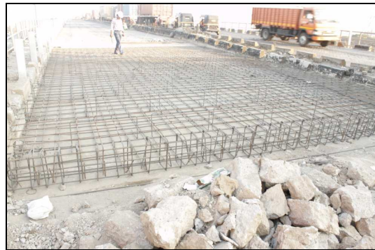
Fig.15 Slab Casted at the site over the bridge at the approach
