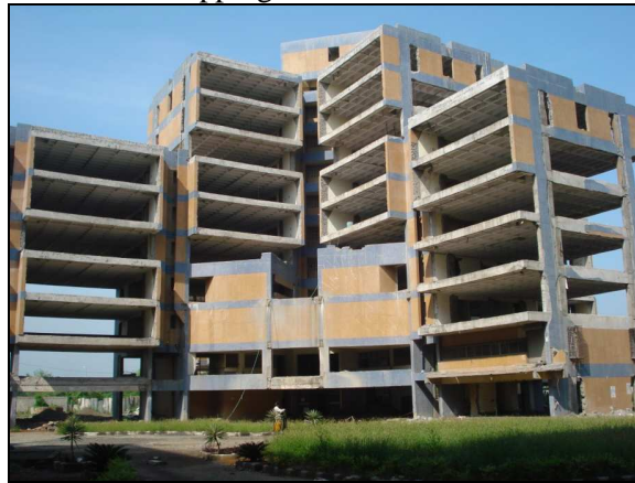
Fig.23 D-block of SEZ Commercial complex
