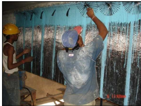
Fig.17 Encasing the girders with Carbon Fiber Wrapping
