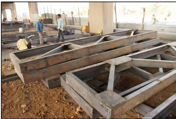
Fig.14 Steel Trusses being fabricated at site
