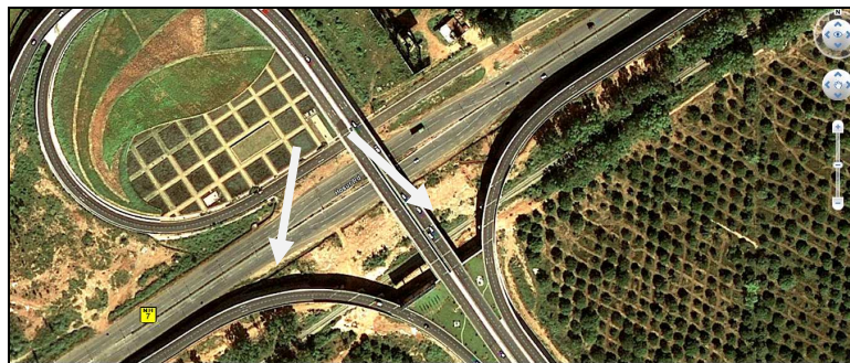
Fig.20 NH 7 Highway Site
