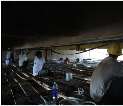
Fig.16 Pre-stressing in process and the finished laminate with anchor plates at end
