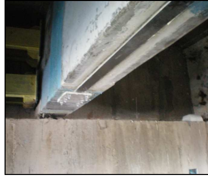
Fig.16 Pre-stressing in process and the finished laminate with anchor plates at end
