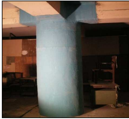
Fig.6 Final look of column after plastering
