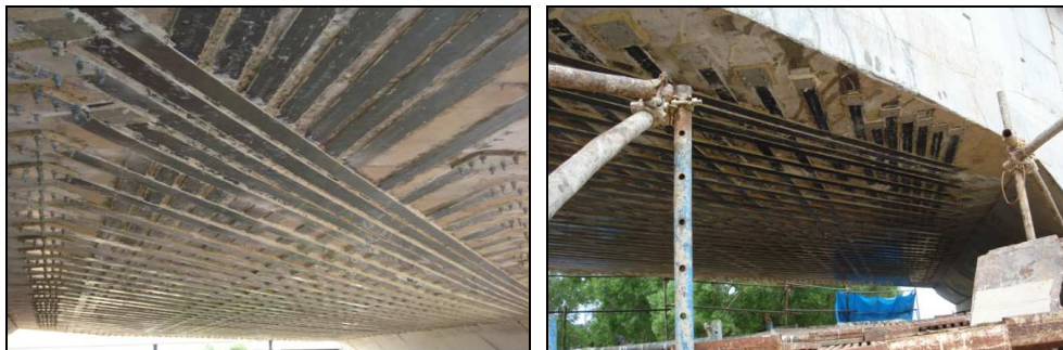
Fig.22 Final view of the two Skew Slab of two Bridges
